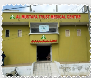
Medical Centre Orangi, Karachi Upgraded in May 2020
