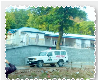
Dispensary Chhajana Kotli Sattian Estb in Sep 2019
